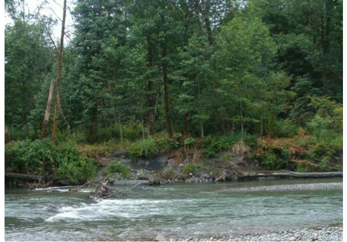
Eroding riverbank before construction
