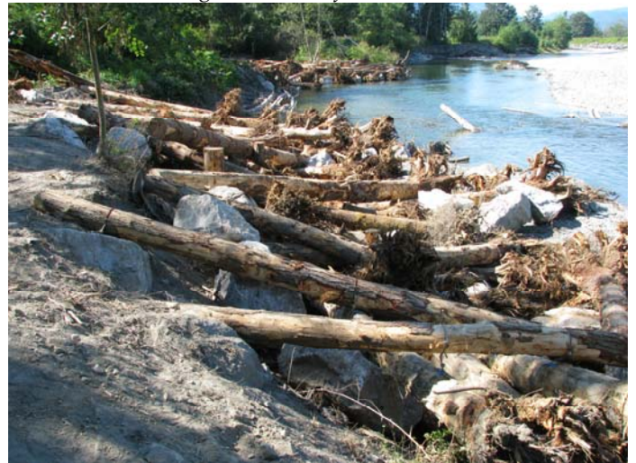
The same location, after construction.
