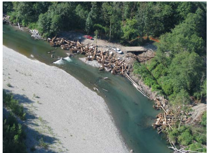
Aerial photo of entire project site
