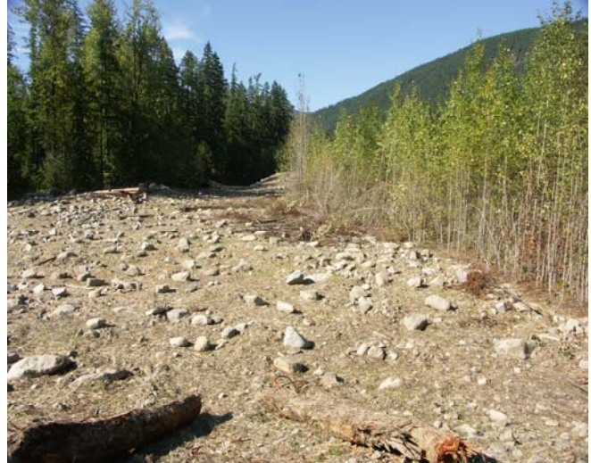
July 2009 Levee removal complete and site reshaped
