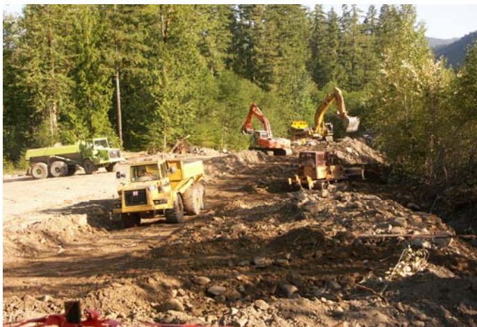
July 2009 Levee removal underway
